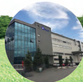
HT Solar Energy J.S.C.
